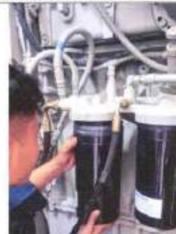
Pemasangan Secondary Fuel Filter Genset CH10931
