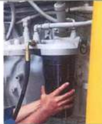
Pemasangan Primary Fuel Filter Genset CH10930
