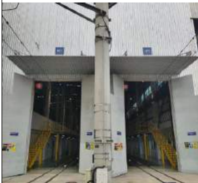
Inspection Shed / Gedung Inspeksi
